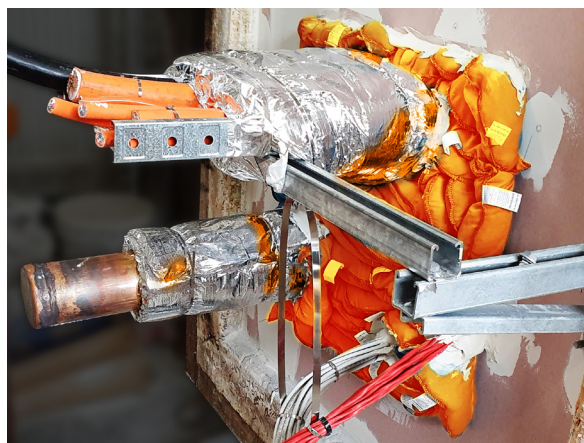
Image: Metal Pipes up to 100mm, unwrapped bundles of small cables and cable trays
